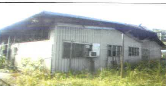
Fig 18.0 View showing Side view of the building.
