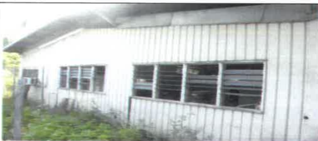
Fig 17.0 View showing external view of the building.
