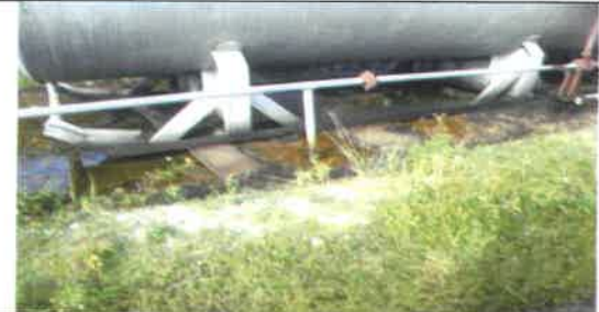
Fig 34. 0 View showing old waste tank to be inspect by PPL Safety officer.
