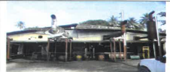
Fig 26. 0 View showing front view of the Power house.
