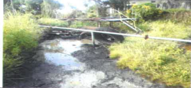
Fig 33.0 View showing no proper waste tank to stored oil.
