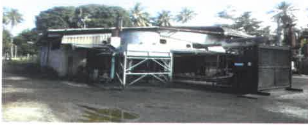
Fig 29.0 View showing side view of the building
