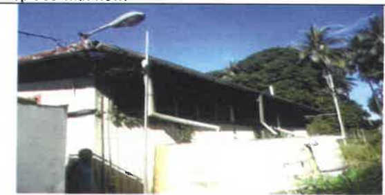
Fig 12.0 View showing side view of the building.
