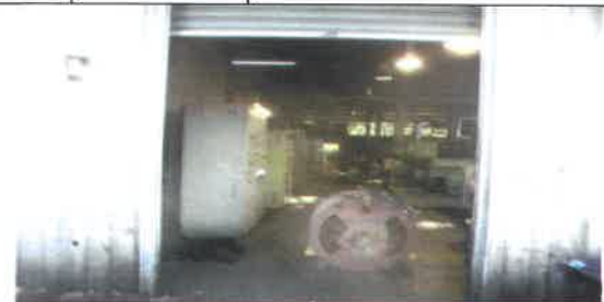
Fig 32.0 View showing old gate frame to be remove and reconstructed with new.
