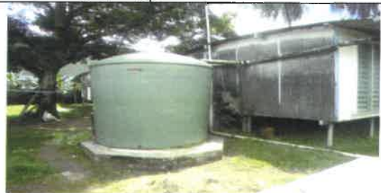
Fig 12.0 View showing old fibro sheets to be remove and install new panel rib sheets.
