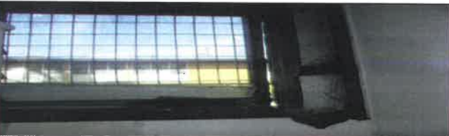
Fig 15.0 View showing wore insect screen to be remove and replace with new.
