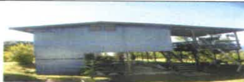
Fig 5.0 View showing external view of the building.
