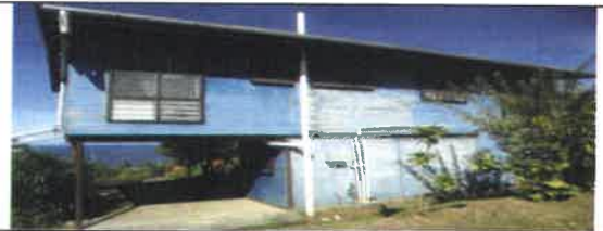
Fig 2.0 View showing external view.
