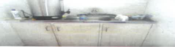
Fig 25.0 View showing mini Kitchen to be fabricated with new frame.
