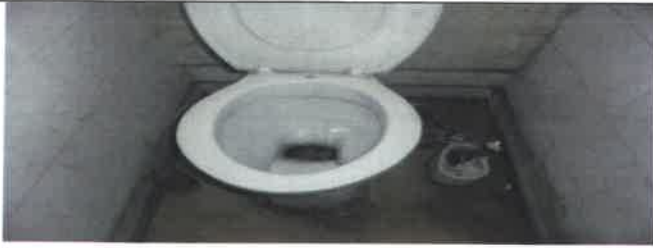
Fig 29.0 View showing faulty toilet pot to be remove and replace with new.
