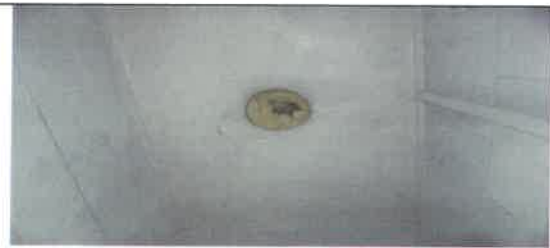
Fig 30.0 View showing faulty light frame to be remove and replace with new.
