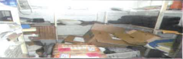
Fig 23.0 View showing poor ventilation. File section 2 office.
