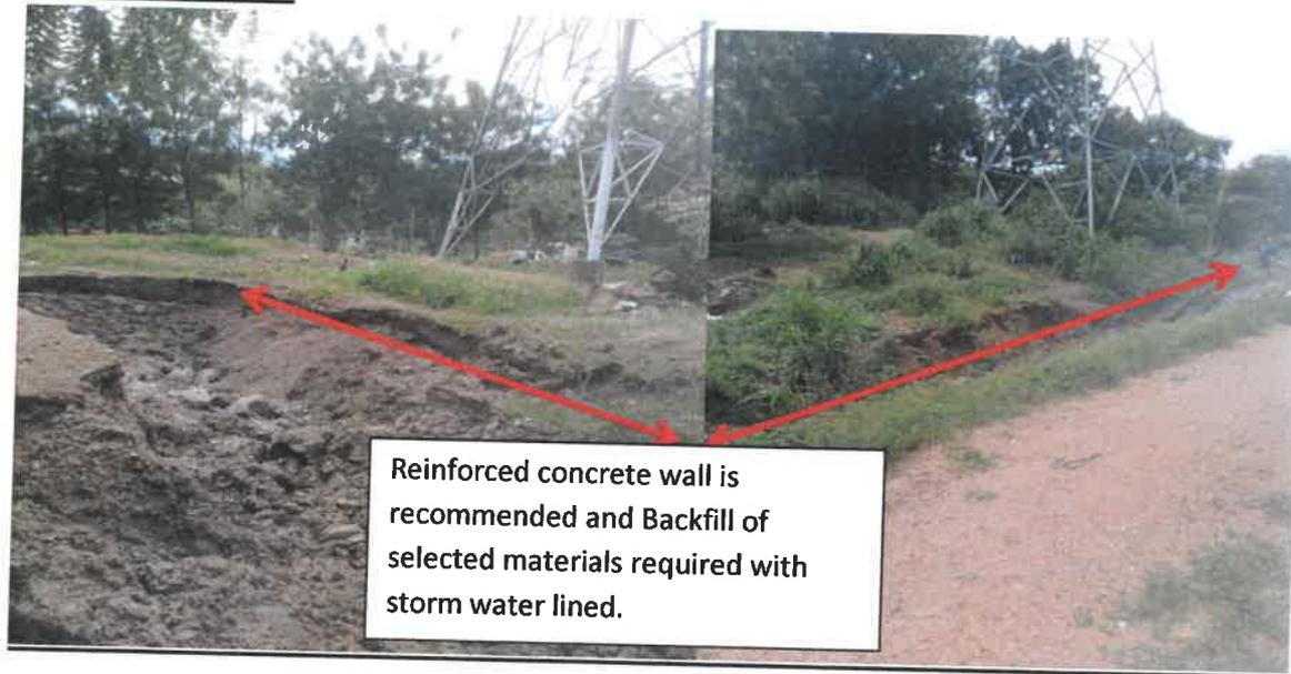
Reinforced concrete wall is recommended and Backfill of selected materials required with storm water lined.
