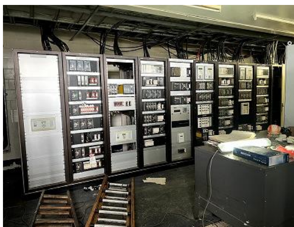
Figure 2: Substation control room in need of renovation
