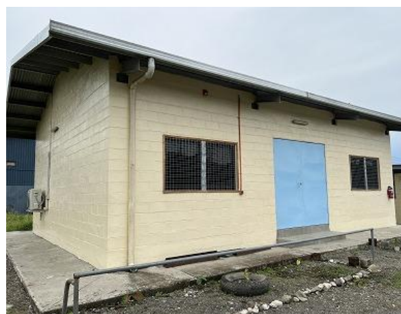
Figure 3: Example of a newly constructed control building in a substation
